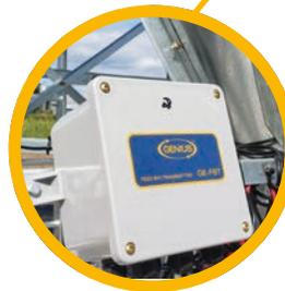
The **GE-FBT/SB** (feed bin transmitter) is connected to the bin load cells
